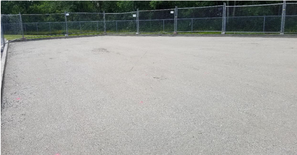
PLAY AREAS SUBGRADE READY FOR ASPHALT
